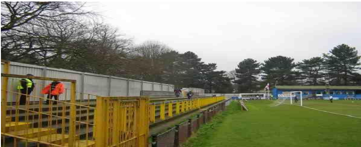
Hatfield Road of East Terrace
