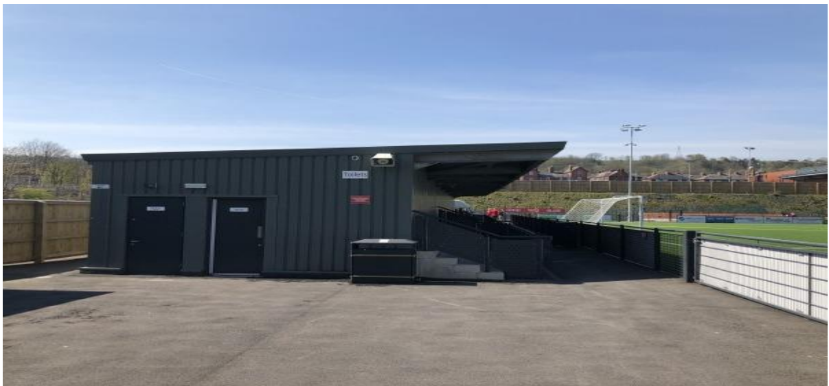
Railway Lane Enclosure
